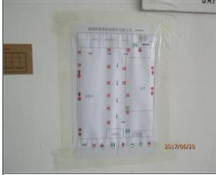
Photo of fire safety equipment Evacuation plan.JPG
