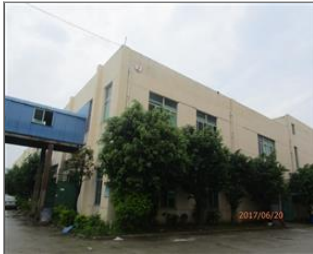
External photo(s) of the production unit(s) No.2 Production building.JPG
