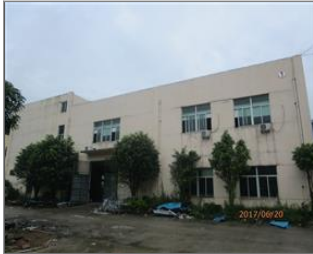
External photo(s) of the production unit(s) No.1 Production building.JPG
